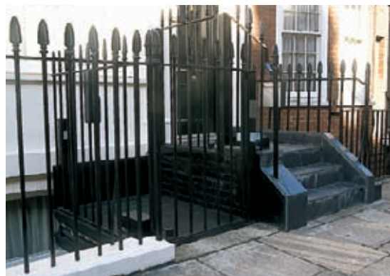
Many entrances to 18th-century and 19th-century terraced town houses have steps up to the front entrance, along with a basement area. An external platform lift was installed within the basement area of this London house, the steps and landing altered and the railings adapted in keeping with the existing design. A lift was installed within the house. The house has since been sold and the platform lift removed.
