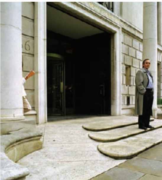
This elegant solution at the Royal Institute of British Architects overcomes a small change of level at the entrance.
