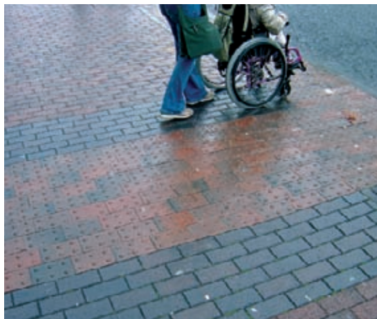
In Tunbridge Wells, where the paving tradition is red and blue brick, the tactile surface at crossings is made with brick paviors.
